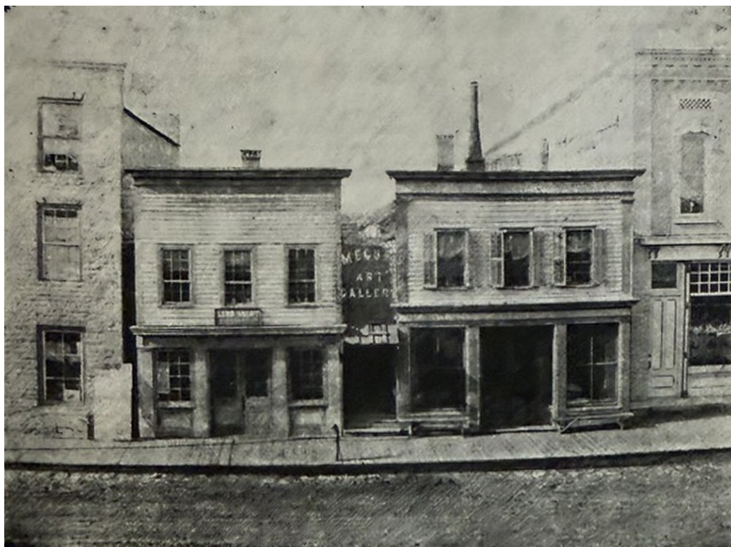
Megow building and adjoining structures prior to the time that third story was added on. (Megow photo)
